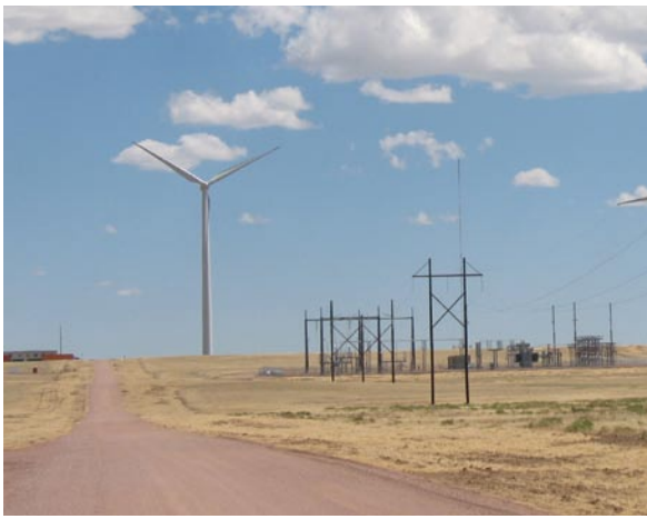
Fig. 2: Towers begin dotting the landscape at the Cedar Point Wind Farm.
