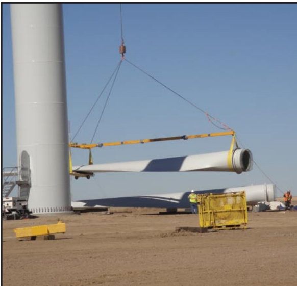
Fig. 6: Blades are lifted into place at the Cedar Point Wind Farm.
