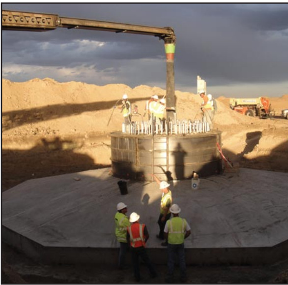
Fig. 4: Foundations being poured at Cedar Point.
