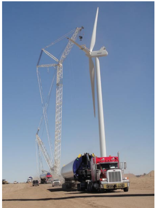
Fig. 3: Tower sections are delivered to the construction site.
