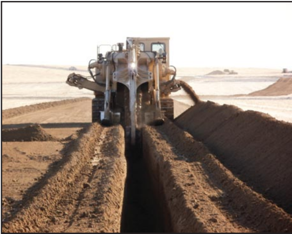
Fig. 5: Trenching begins, connecting turbines to the grid.
