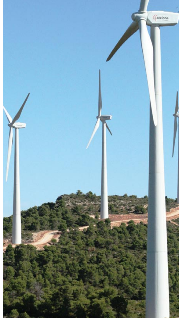
Fig. 1: In operation since 2008, the Losilla Wind Farm in Spain features 16 towers of 80 m supporting an AW-1500 wind turbine.
