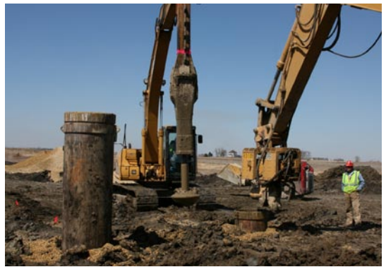
Fig. 3: Turbine excavation reinforced and prepared for foundation construction.
