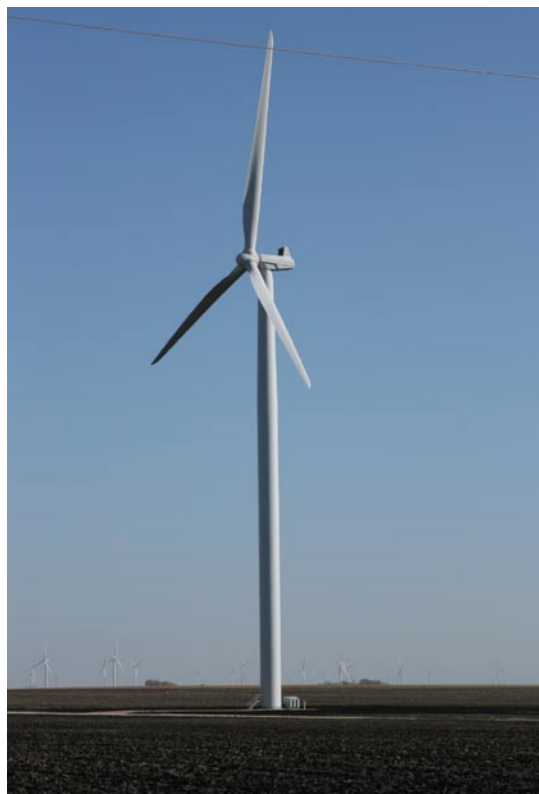
Fig. 5: RAP supported turbine.
