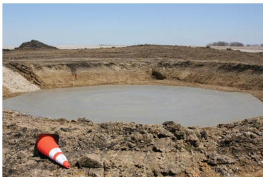
Fig. 4: Foundation excavation proceeds.
