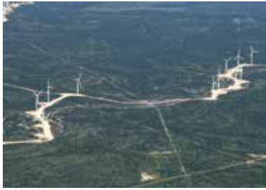
Forest Creek Wind Farm near Big Spring, Texas.
