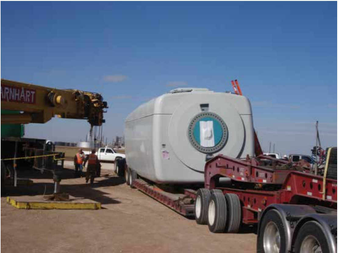
Figure 4: Nacelle being delivered and readied for unloading.
