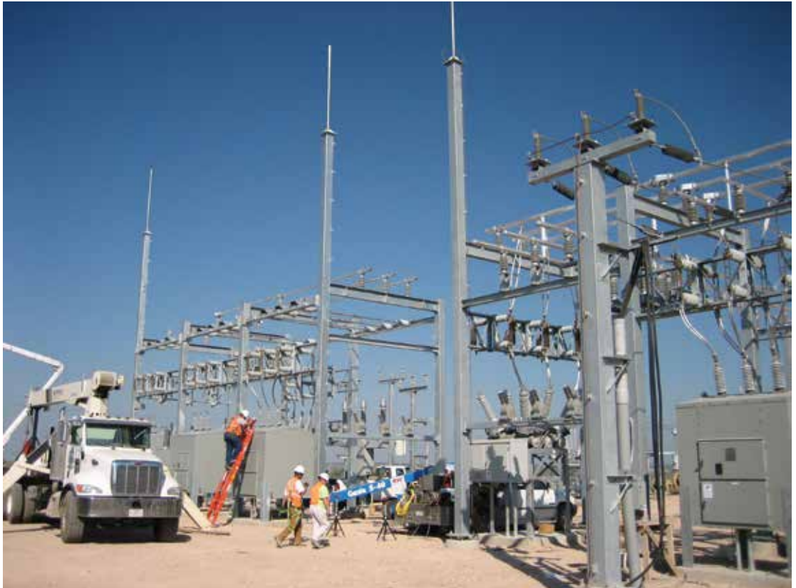
Figure 6: Crews nearing completion of substation work.
