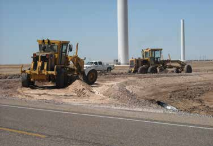
Figure 5: Graders remove the turning radius after deliveries are completed.
