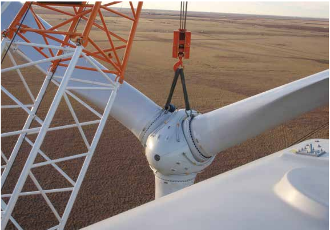
Figure 2: A rotor is lifted into position for installation onto the nacelle.
