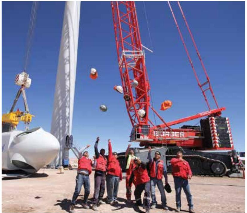
and owner of Gruas Burger. “We are very experienced in erecting wind turbines, so we offered the developing company our services with the NT crane so they only needed to build 5.5-meter-wide roads for the crane instead of 10 meters, which is usually needed for a crawler crane. We helped them save a significant amount of money.”
