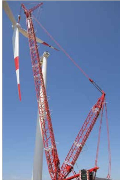
ments. Equipped with its narrow track chassis, the CC 2800-1 NT can be driven from one construction site to the next, even when access is tight, while fully rigged with counterweights, 334.6 ft. (102 m) main boom and LF 2 fixed jib, saving precious time and increasing productivity.
