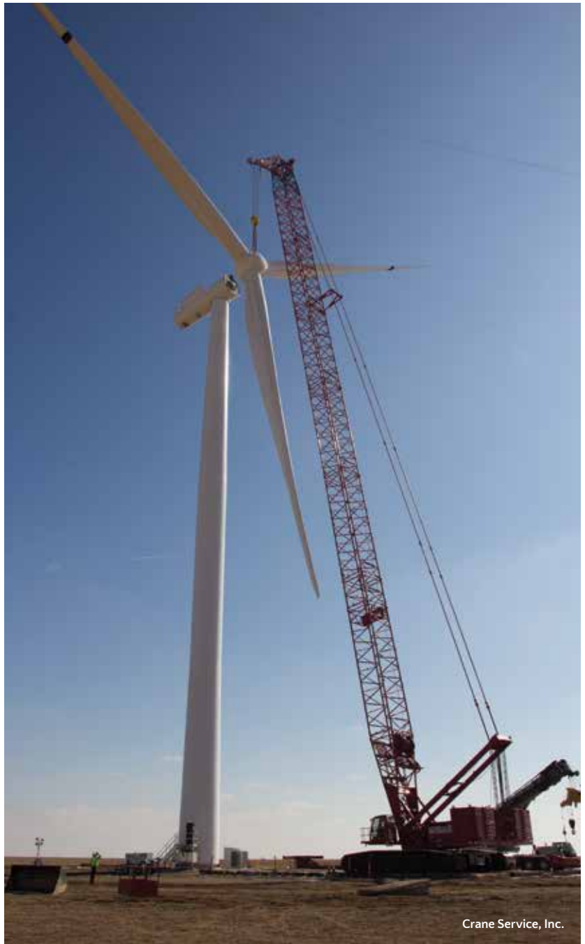
The Manitowoc 16000, a 440-ton crawler crane, hoists a wind turbine rotor in a wind park in northern Texas. The rotor, hub, and blades weigh around 95,000 pounds.
