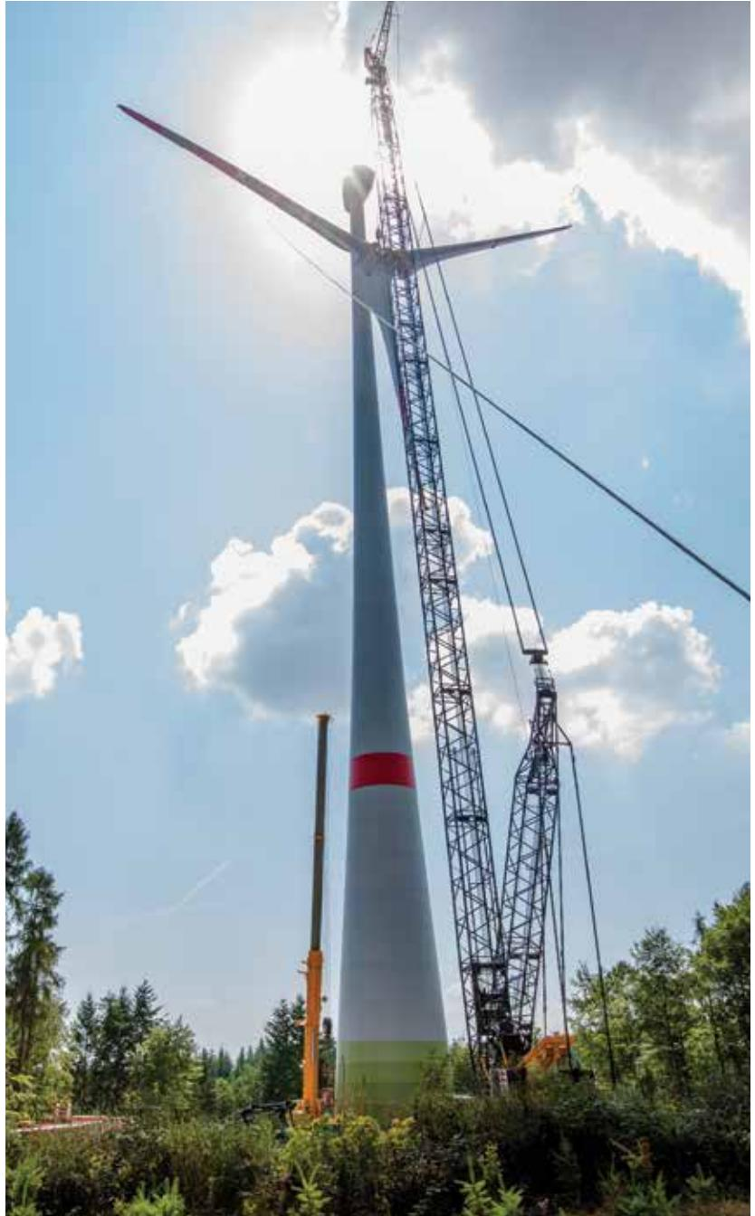
for the task at hand. This configuration enabled it to safely handle the three main lifts required to erect the wind turbine, which had a hub height of 130 meters, while working with working radii of 20 to 22 meters. The team estimated a total of three days for the work: On the first day, The CC 2800-1 crawler crane lifted the 52.9-ton
